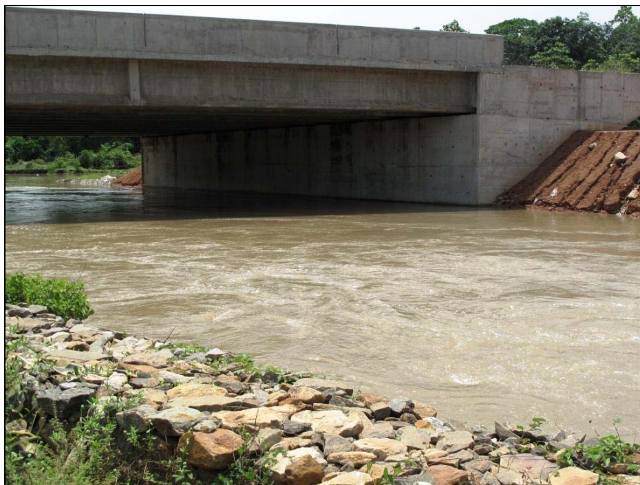
Flood mitigation measure at the JICA section
