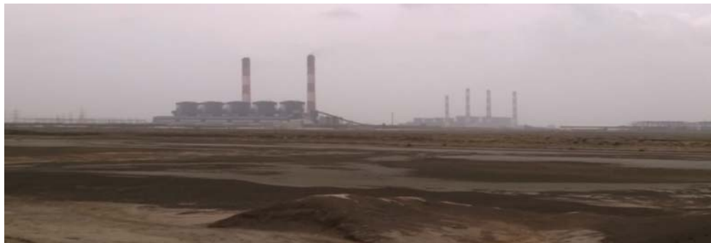
Figure 4: Location of TATA Mundra Power Project and Adani Power Project
